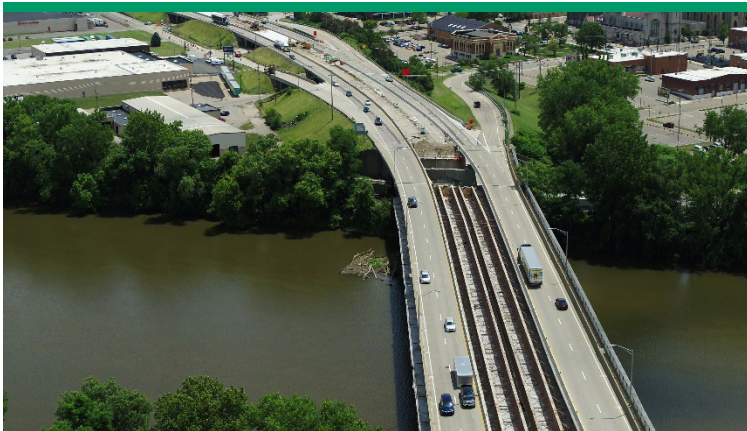
Reconstruction of I-70 through Zanesville between U.S. 40 and State Route 93 includes four phases. This $88 million project includes a complete rebuild of the interstate and overpasses through Zanesville. The project, which began in Summer 2021 is scheduled for completion in Fall 2027.
