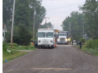
Twinsburg Township Heights Allotment Rd Reconstruction
