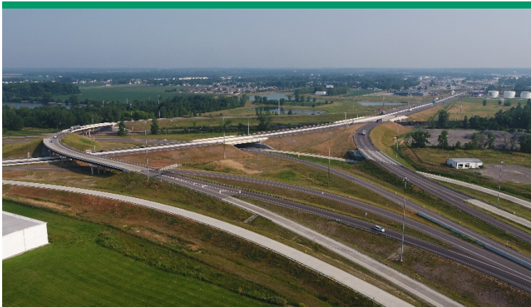
Reconstruction of five miles of I-75 through Findlay included replacing all mainline bridges on I-75, the Harrison Street overpass, redesigning and reconstructing the interchanges between U.S. 68/State Route 15 and Interstate 75 and with U.S. 68/State Route 15 at Lima Avenue. The $114 million project was completed in Fall 2020.
