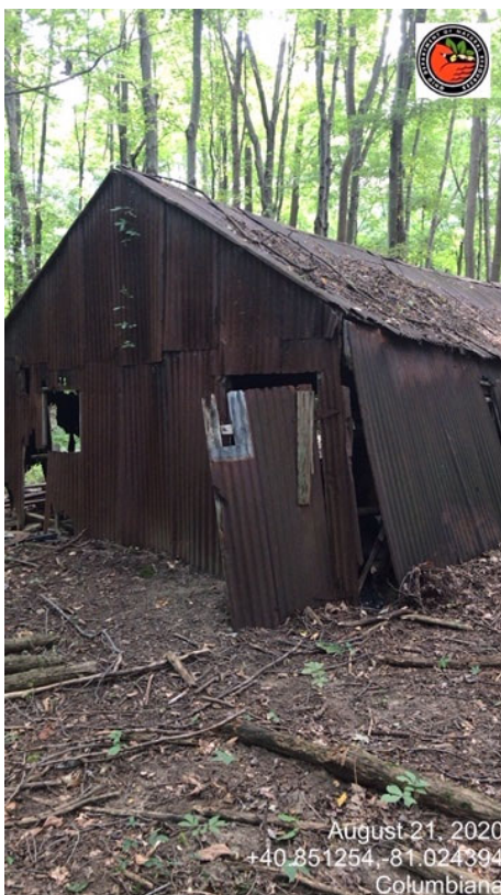
Columbiana #3 Project, Outside Powerhouse
