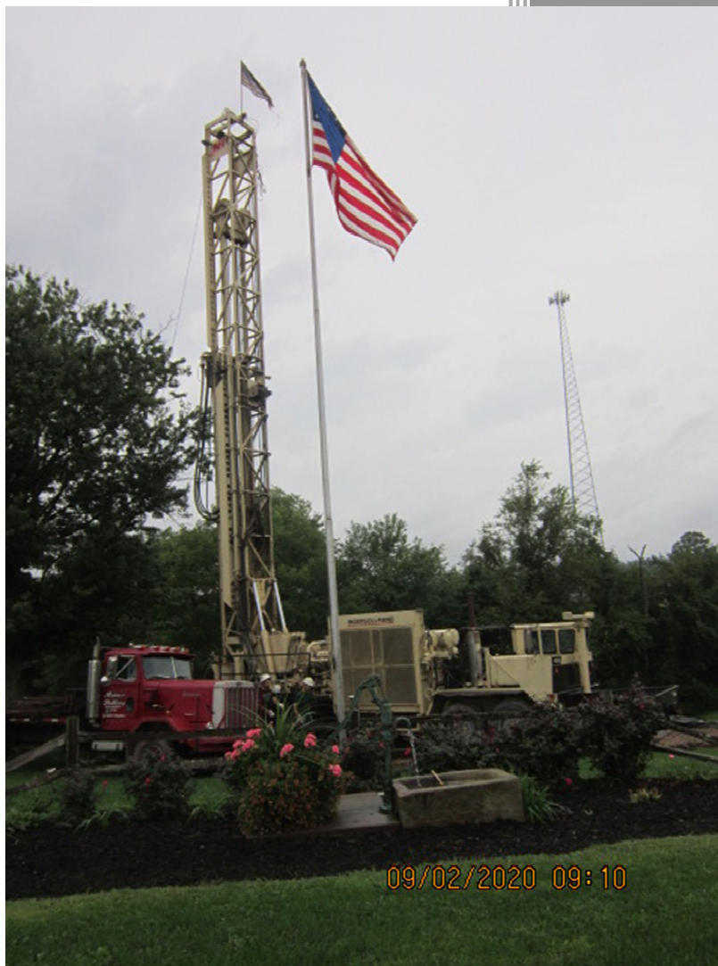
Monroe #1 Project, Gardner #1 Well, Plugged September 2020
