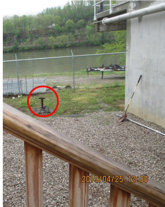
Washington #8 Project, Newport Sewer & Water #1 Well
