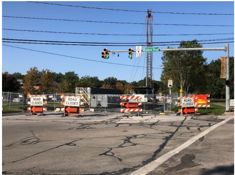
Cuyahoga #9 Project, Wolf Road #1
