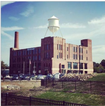
The Joseph & Feiss Co. facility in Cleveland was redeveloped into the Menlo Park Academy.
