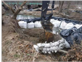
Middle Fork Little Beaver Creek Excavation
