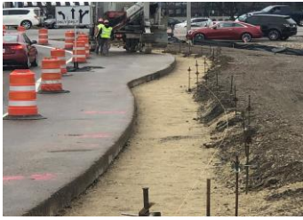
Montgomery County TID- Miami Township Lyons Rd Pedestrian Access
