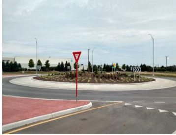
Village of West Jefferson- SR29/US40 Improvements
