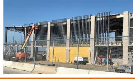
Akron-Canton Regional Airport Authority- Gate Expansion
